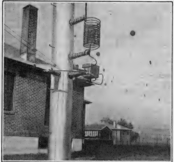
FIG. 284.—Antenna loading coil and ammeter—Station KDKA.
