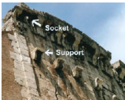
The supports are visible in this picture
