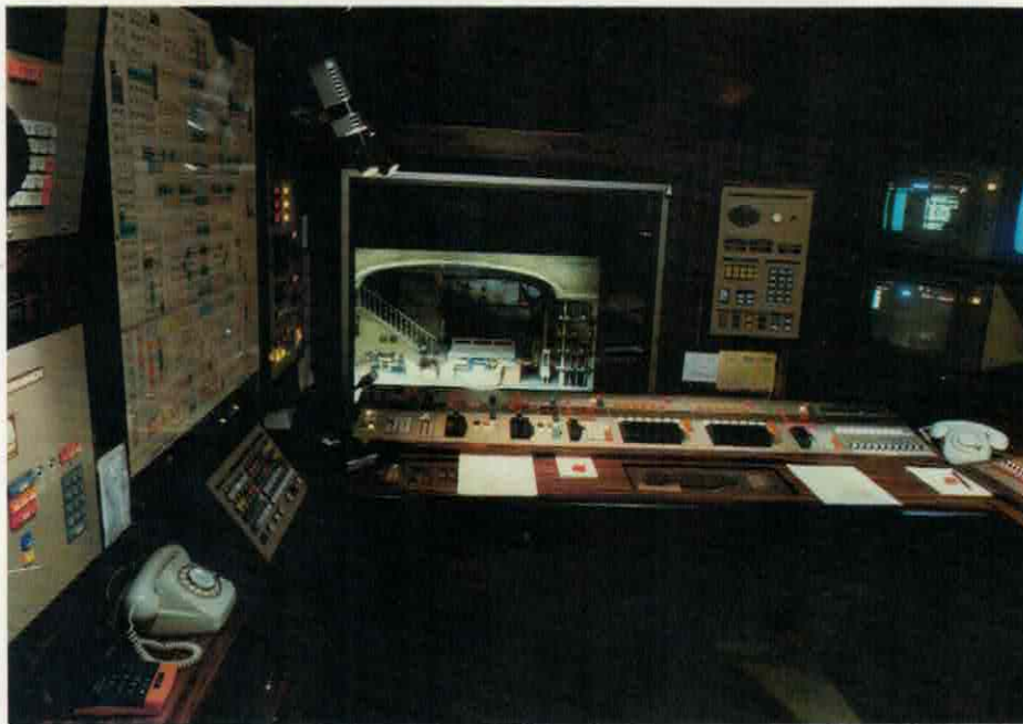
Strand Lighting in Vienna - installed by Ludwig Pani. Above: the Galaxy system at the Vienna State Opera (also in view, extreme left, is the Pani PEF-M remote control for motorised spotlights). Right (top): A Galaxy at the Theater in der Josefstadt. Right (lower): A Light Palette at the Volkstheater.
