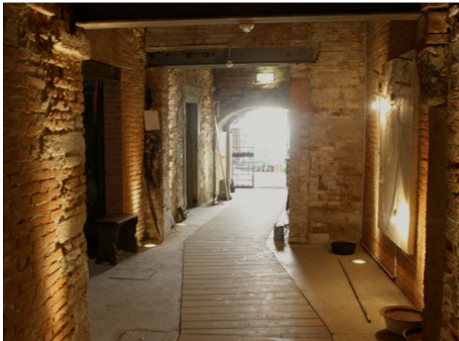
Plate 12 Ground floor path from la porta d'acqua to the courtyard, (added security lighting). Palazzo Fortuny. Photo Zeke Smith.
