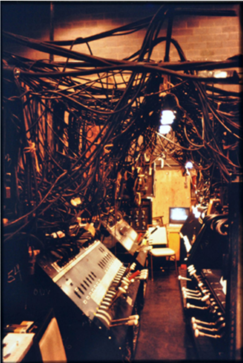
Piano board installation, Washington 1977 Klavierbrett-Installation, Washington 1977
