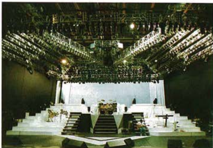
The lighting rig installed at The Marquee club in London.
