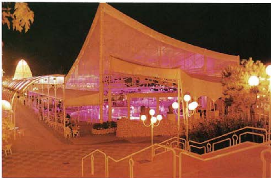
The Summer disco - open-sided with a vaulted tubular structure and sculptured PVC tarpaulin cover.
