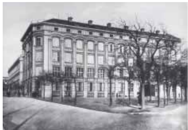
OSRAM Fábrica de Lámparas in Madrid, Spain was founded in 1914 by the Deutsche Gasglühlicht-Aktiengesellschaft with the involvement of Siemens and AEG.
