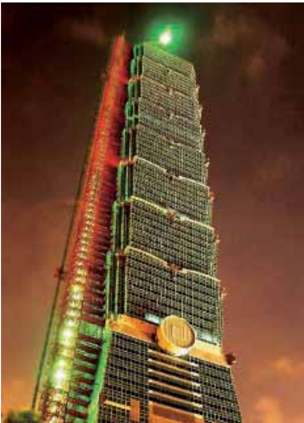
At 508 metres, "Taipeh 101" is the tallest structure in the world. Osram was chosen as a system supplier to provide the lighting equipment.
