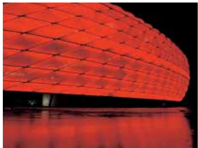
Thanks to more than 25,000 fluorescent lamps and 12,000 ECGs from OSRAM installed in Siteco luminaires, the Allianz Arena in Munich looks splendid in white, blue or red light
