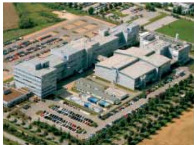
The most advanced optical chip factory in the world is located in Burgweinting near Regensburg. For OSRAM its construction was a milestone in its transition to a high-tech company in the lighting industry.
