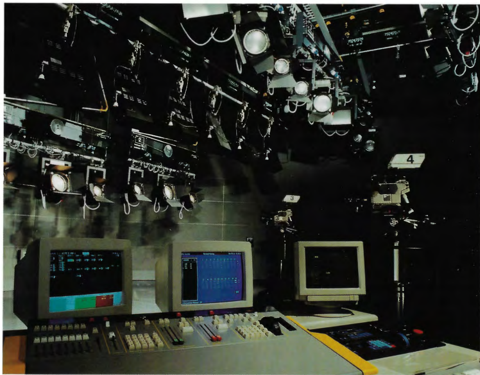
■ The Gemini 2 control desk and an impressive battery of luminaires in the Dr. Straube studio.
