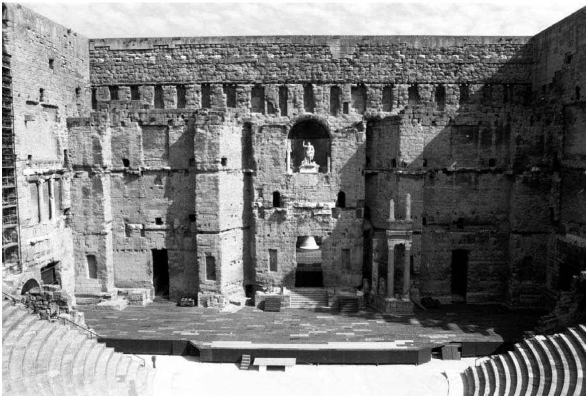
67. Arausio (Orange), theatre. Scaenae frons , showing the three-storey columnnatio and the 19 beam slots for the roof over the stage
