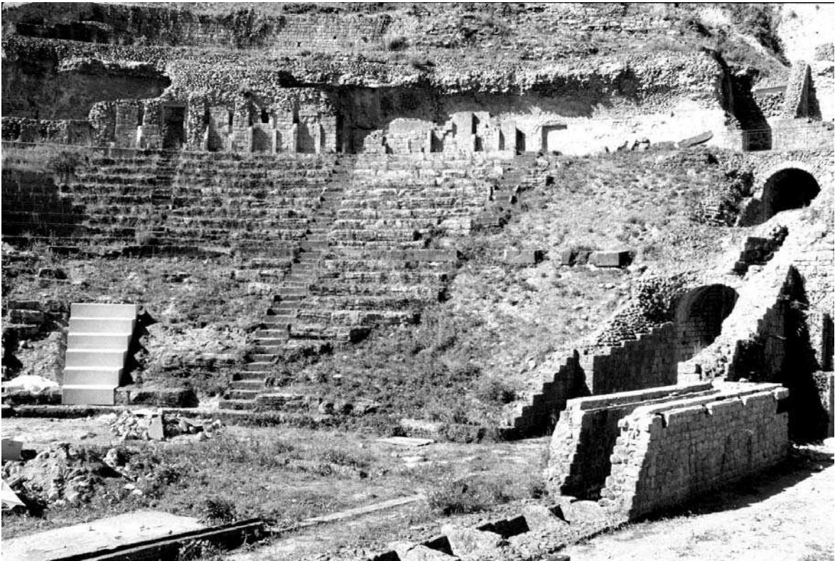
35. Volterrae (Volterra). Cavea looking south, showing part of the proscaenium wall and auleum slot. On extreme right is the west aditus maximus with remains of the tribunal above
