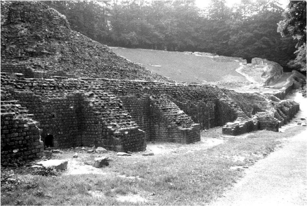
56. Germanicomagus (Saint-Cybardeaux, Bois des Bouchauds), Gallo-Roman theatre. View of buttressed rectilinear wall on north-east side of cavea
