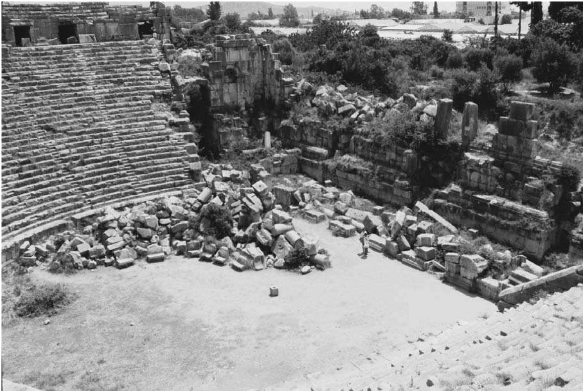
127. Myra (Demre, Turkey), theatre. 1st quarter 3rd cent. AD. Cavea, orchestra, and scene building, looking south-east
