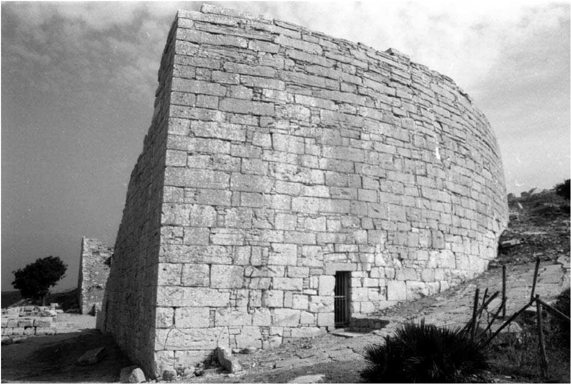
46. Segesta, theatre. Retaining wall around north-west corner of cavea
