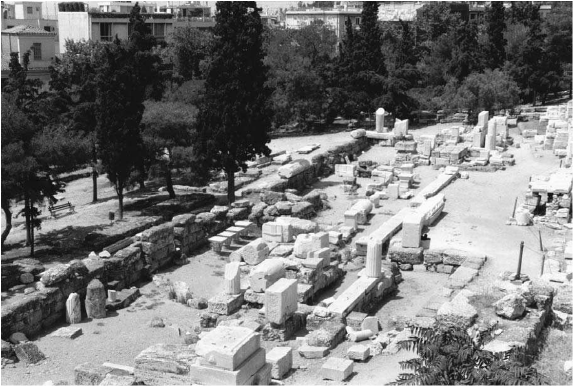
138. Athens, Theatre of Dionysus. View of scene building looking south-west. Parts of the Lycurgan and 2nd cent. BC skene are visible as well as elements from the Neronian scene building
