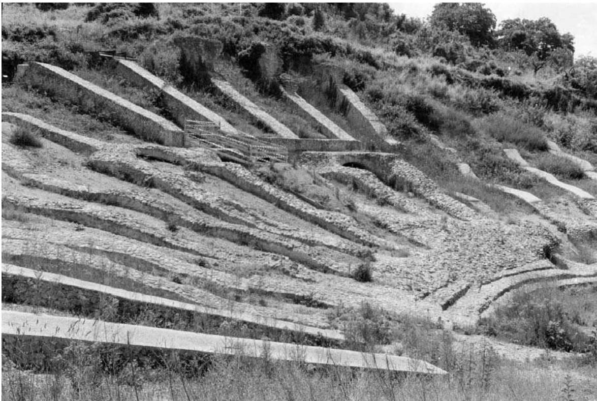
23. Asculum (Ascoli Piceno), theatre. Augustan. Radial substructures under the cavea
