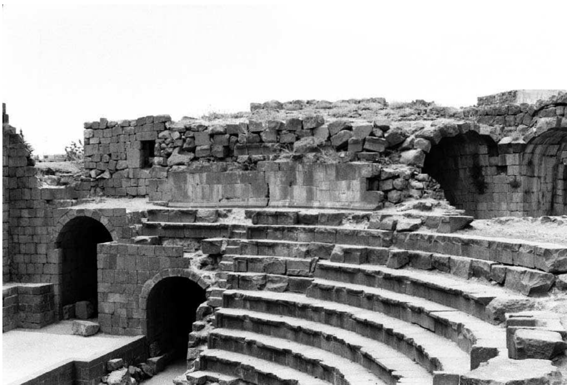
110. Philippopolis (Chabha, Syria), odeum. AD 244-9. View of north side of cavea, showing (left) entrance to the side of the stage; (towards the centre) the west aditus maximus ; (right) the rising gallery under the summa cavea
