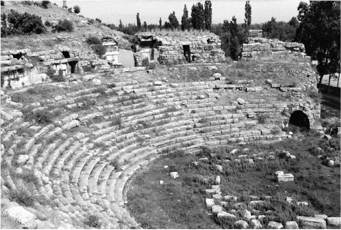
126. Limyra (Dernek, Turkey), theatre. View of the cavea looking south-east. The summa cavea rests upon a vaulted gallery
