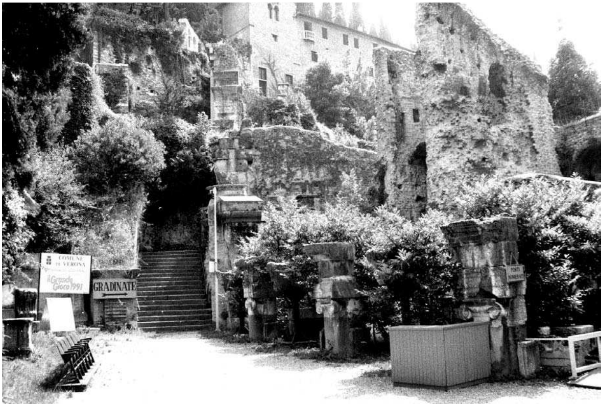
39. Verona, theatre. View of façade and radial substructures on west side of cavea
