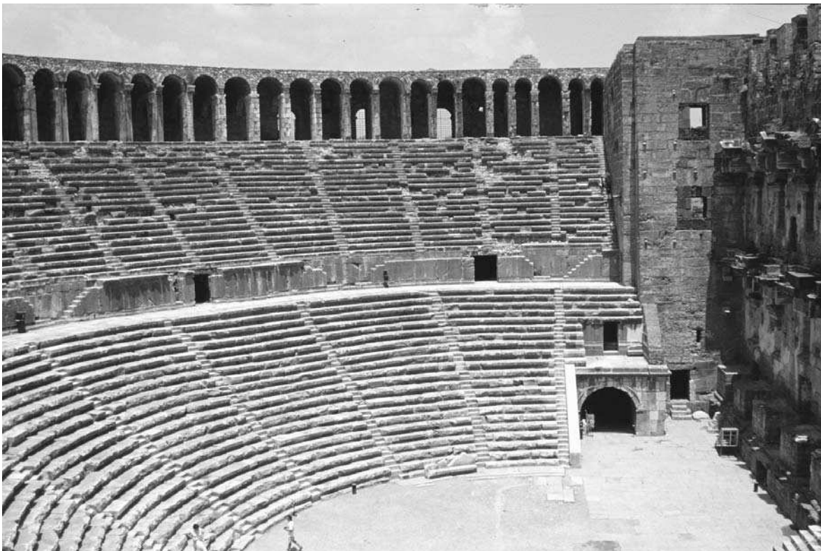
123. Aspendus (Belkiz, Turkey), theatre. Cavea, orchestra, and scene building, looking north. The north tribunal is visible above the north aditus maximus . Nothing survives of the stage
