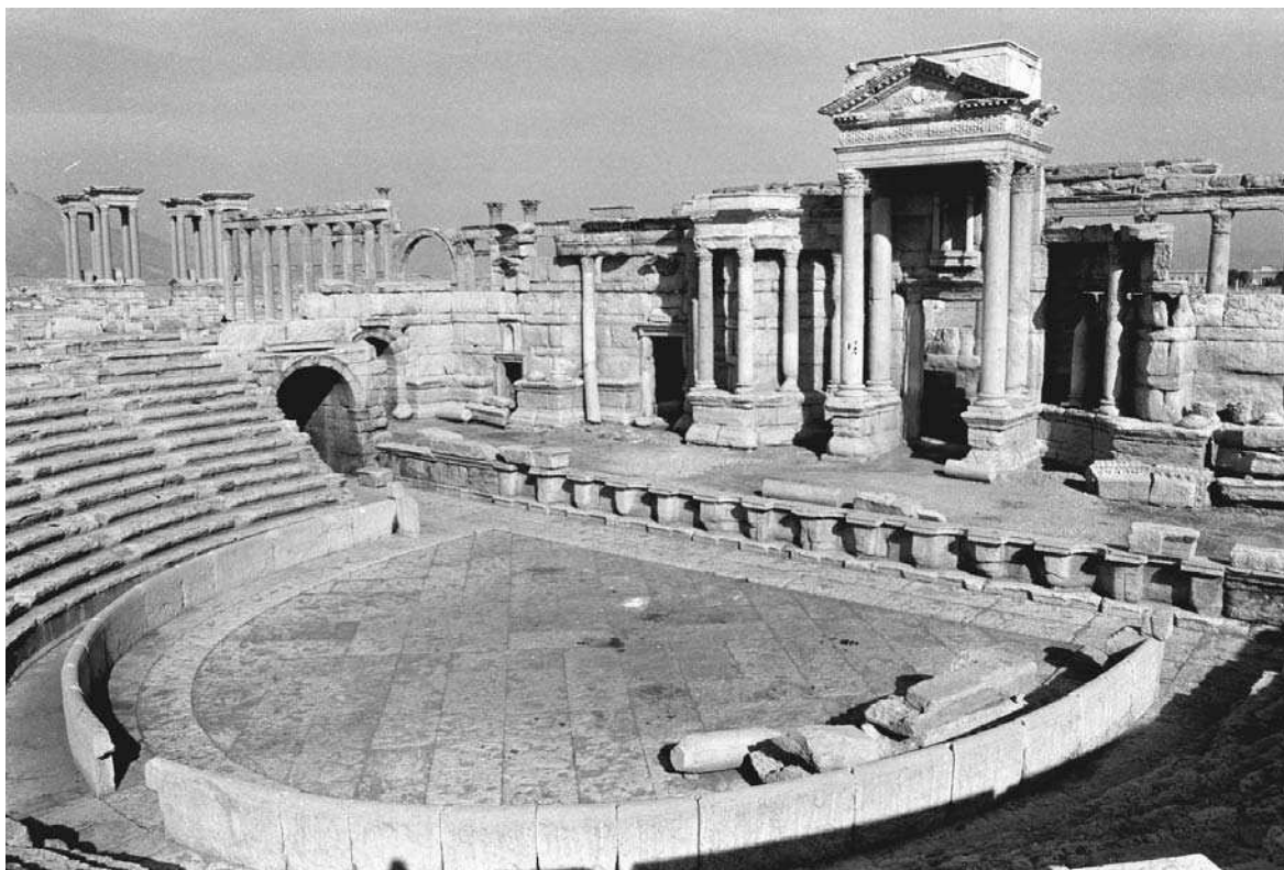
111. Palmyra (Tadmor, Syria), unfinished theatre. 2nd cent. AD. Cavea, orchestra, and scene building, looking north
