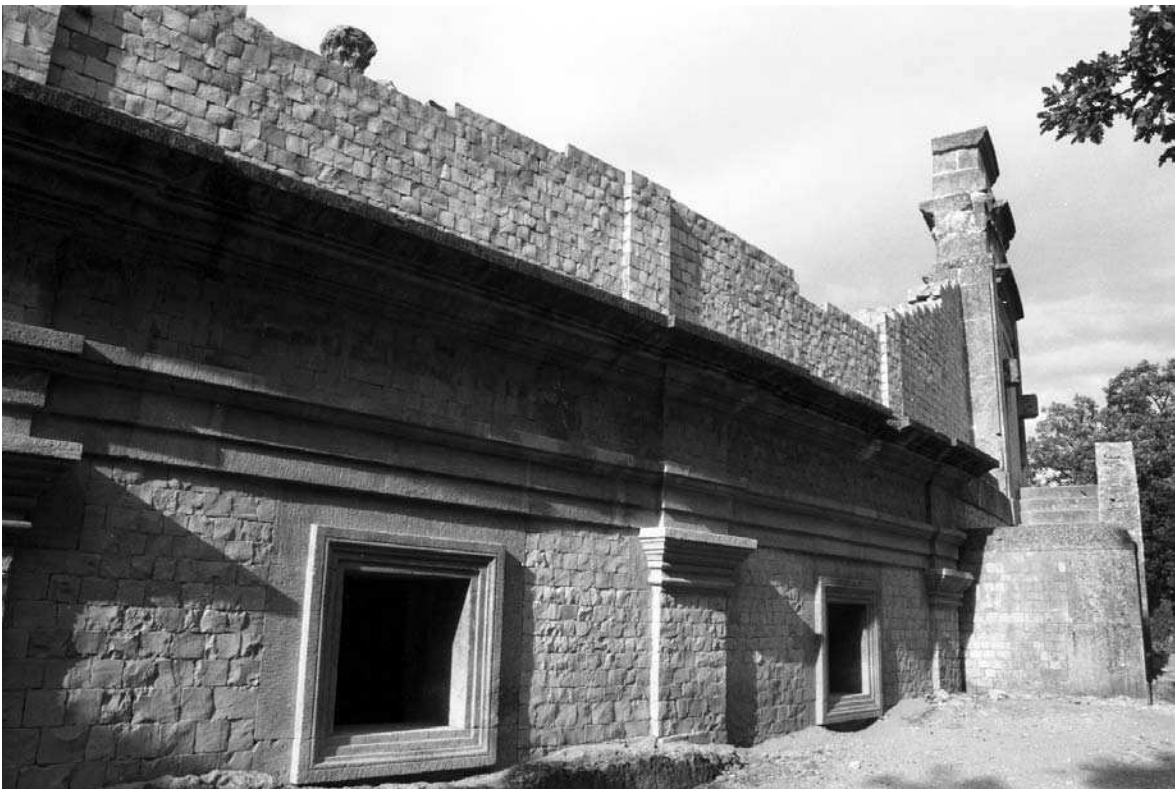
75. Vasio Vocontiorum (Vaison-la-Romaine), theatre. Outer façade, with (right) the staircase leading up to the doorway into the porticus at the top of the cavea . The square windows light the crypta under the porticus
