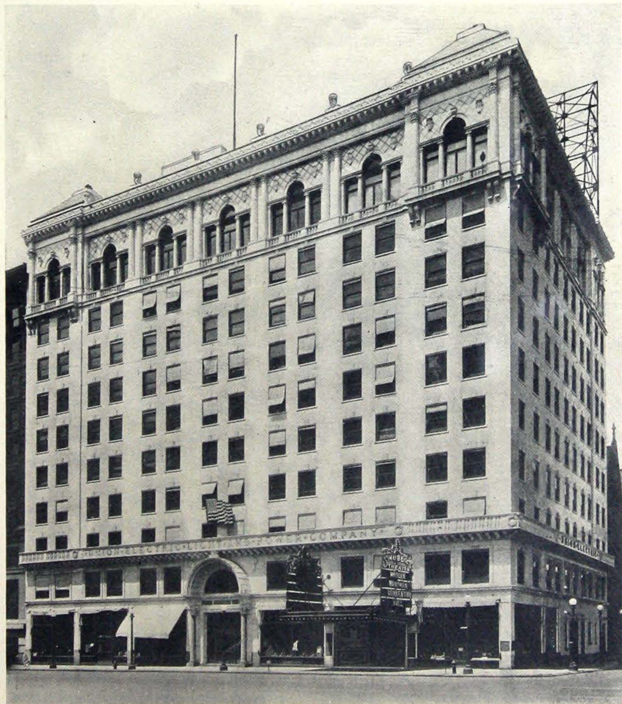
Figure 44—The Shubert-Jefferson, leading dramatic theatre in St. Louis, is equipped with Ward Leonard Vitrohm dimmers.
