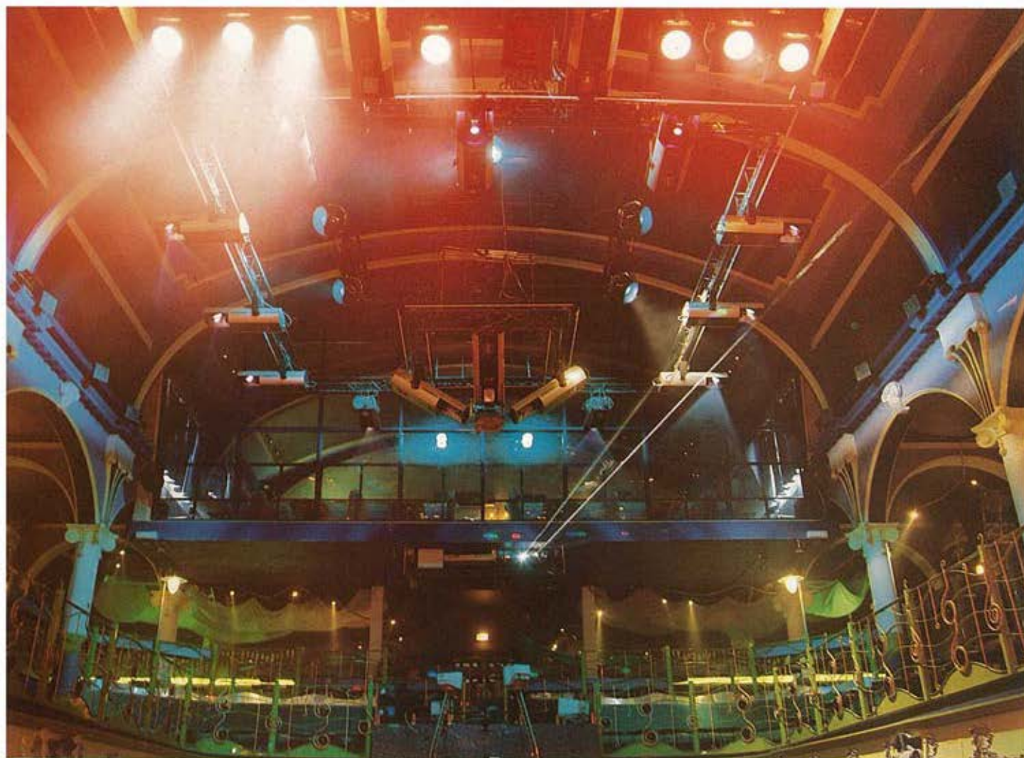
Above the dancefloor of the Forum, Pan Commands and Intellabeams provide the lighting atmospherics, together with an 8W argon laser.
